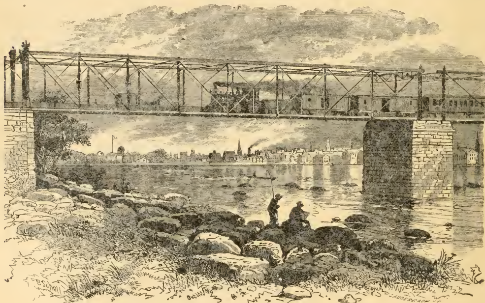
TRENTON—RAILROAD BRIDGE ACROSS THE DELAWARE.
